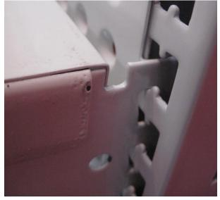
Add the Top Caps. A Single sided end bay has a 945mm Cap; Starter Bay has a 930mm Cap, as does the Last bay on a run of shelving; Add-on bays (middle bays) have a 915mm Cap.
