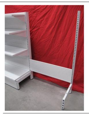
For the Add-on bay – add the 265mm Volcano Panel into the existing post, ensuring that it matches the existing spacing. Attach the other end of the panel to the new post, again, watching the spacing.
